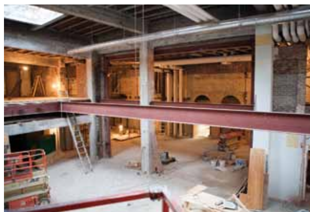
Noel Studio space under construction.
