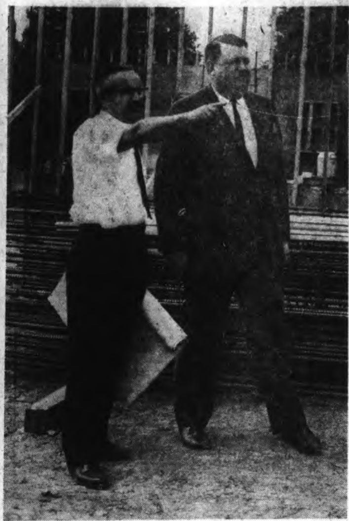
Mr. Conlee, maintenance engineer, points out recent improvements.
