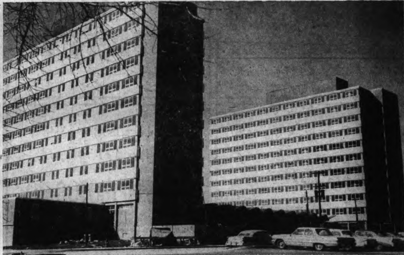
The "Towers" Ready
