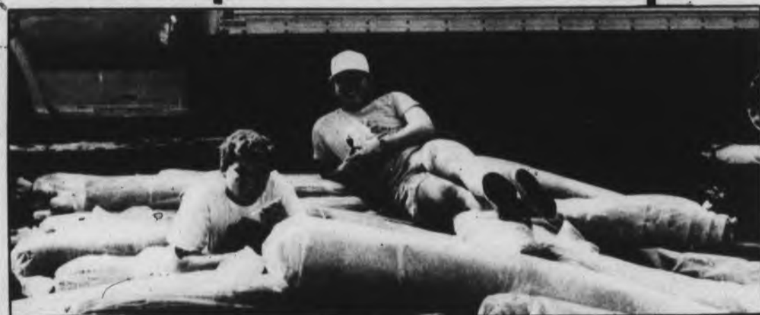
Progress photo/Mike Morris
