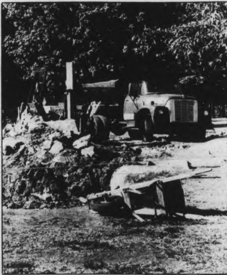
Progress photo/Mike Morris
