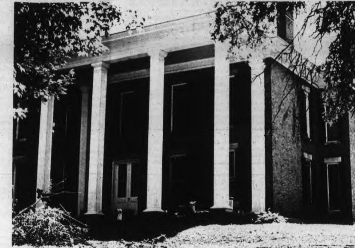
New KA House
