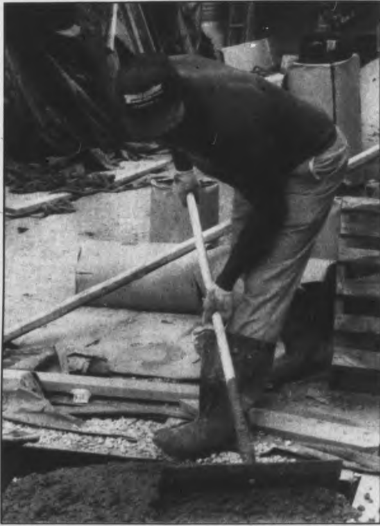
Progress/JAY ANGEL A construction worker pours concrete at the library expansion.
