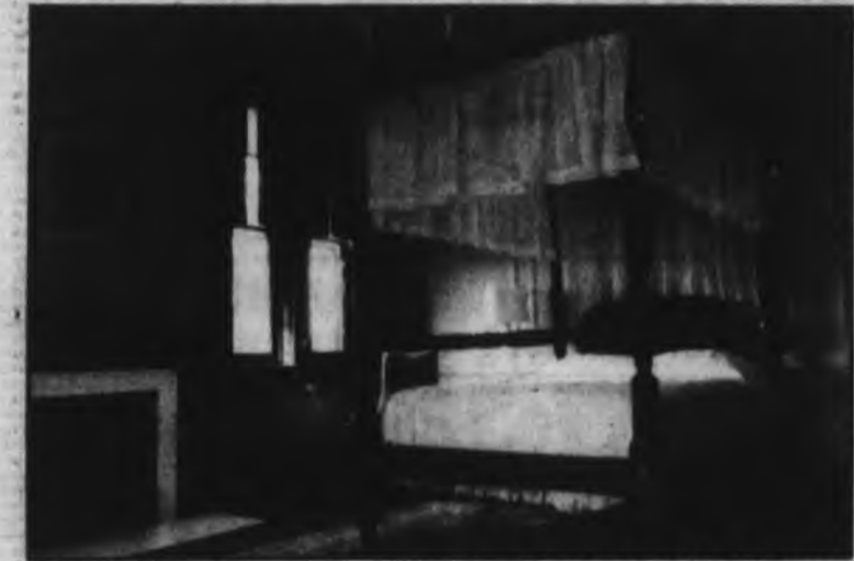
Progress photo/Charlie Bolton
