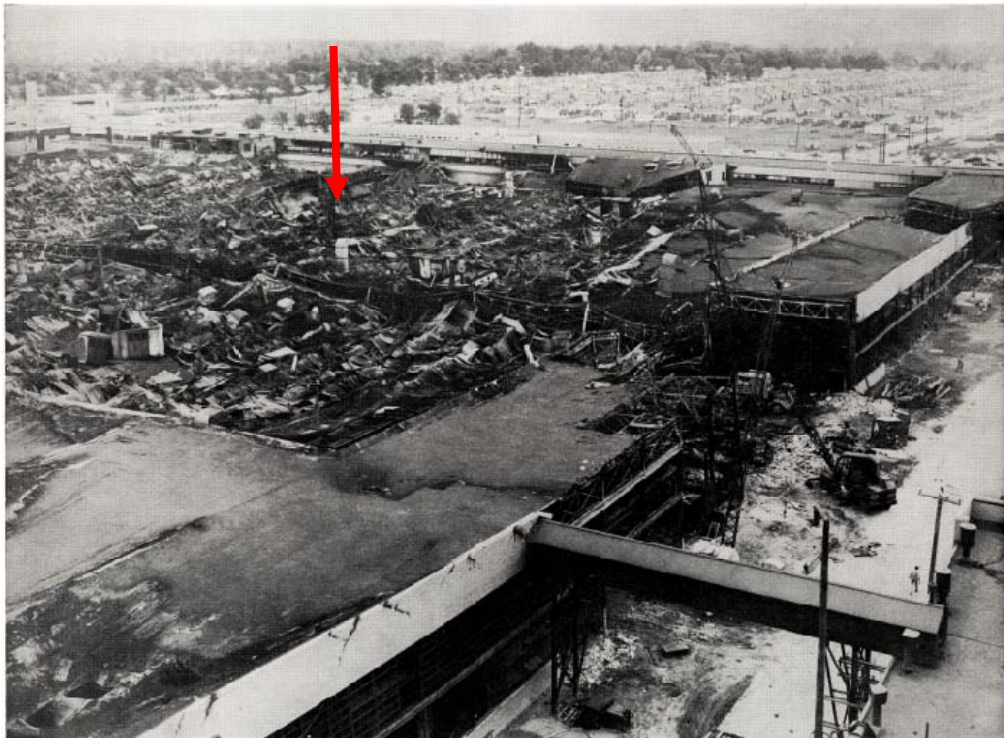
Figure 9: Livonia Transmission Plant Partial Collapse and Confirmed Area of Origin 6
