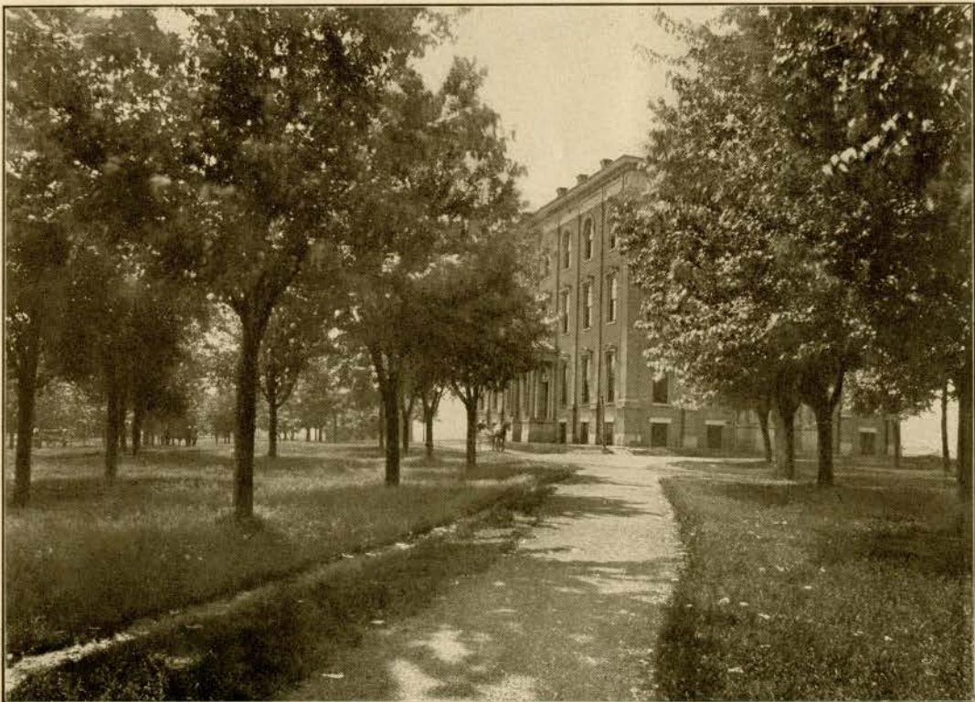
UNIVERSITY HALL AND APPROACH.
