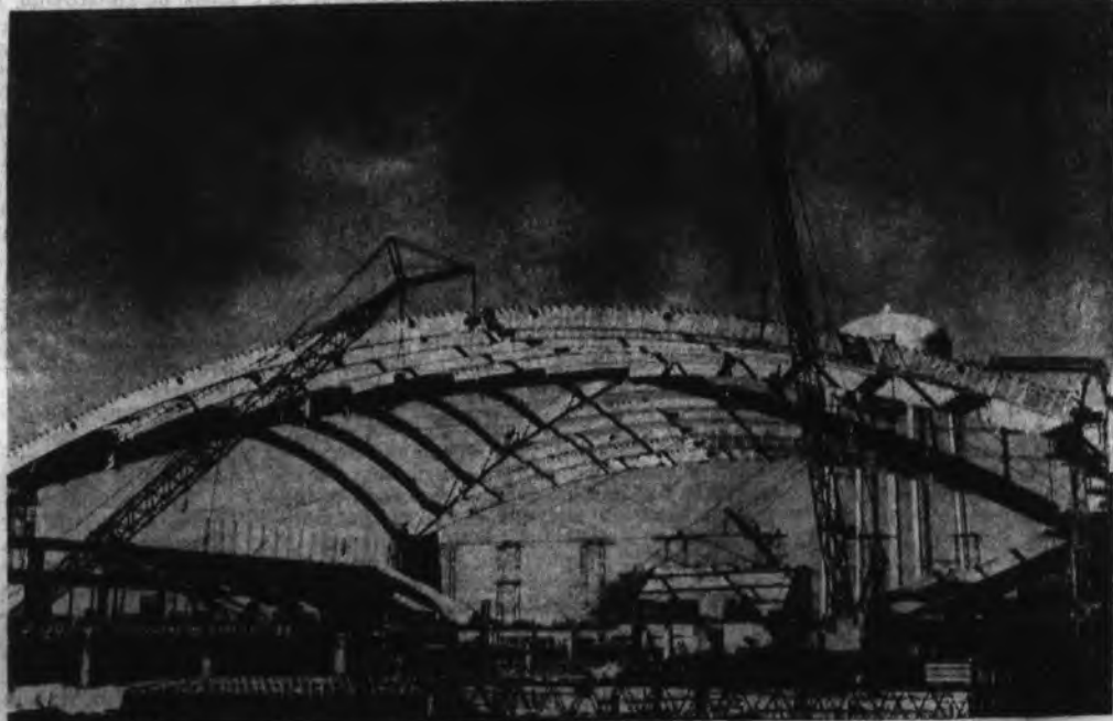
READY FOR THE DECKING . . . With its four main arches, weighing a total of 142 tons, and secondary connecting beams in place Eastern's $3 million Alumni Coliseum awaits the addition of southern pine decking to complete the world's largest roof using a laminated wood structural system. The physical education and athletic plant is slated for completion by April 1, in time for the college's spring commencement to be held in its cavernous auditorium which will seat 7500 for such gatherings.
