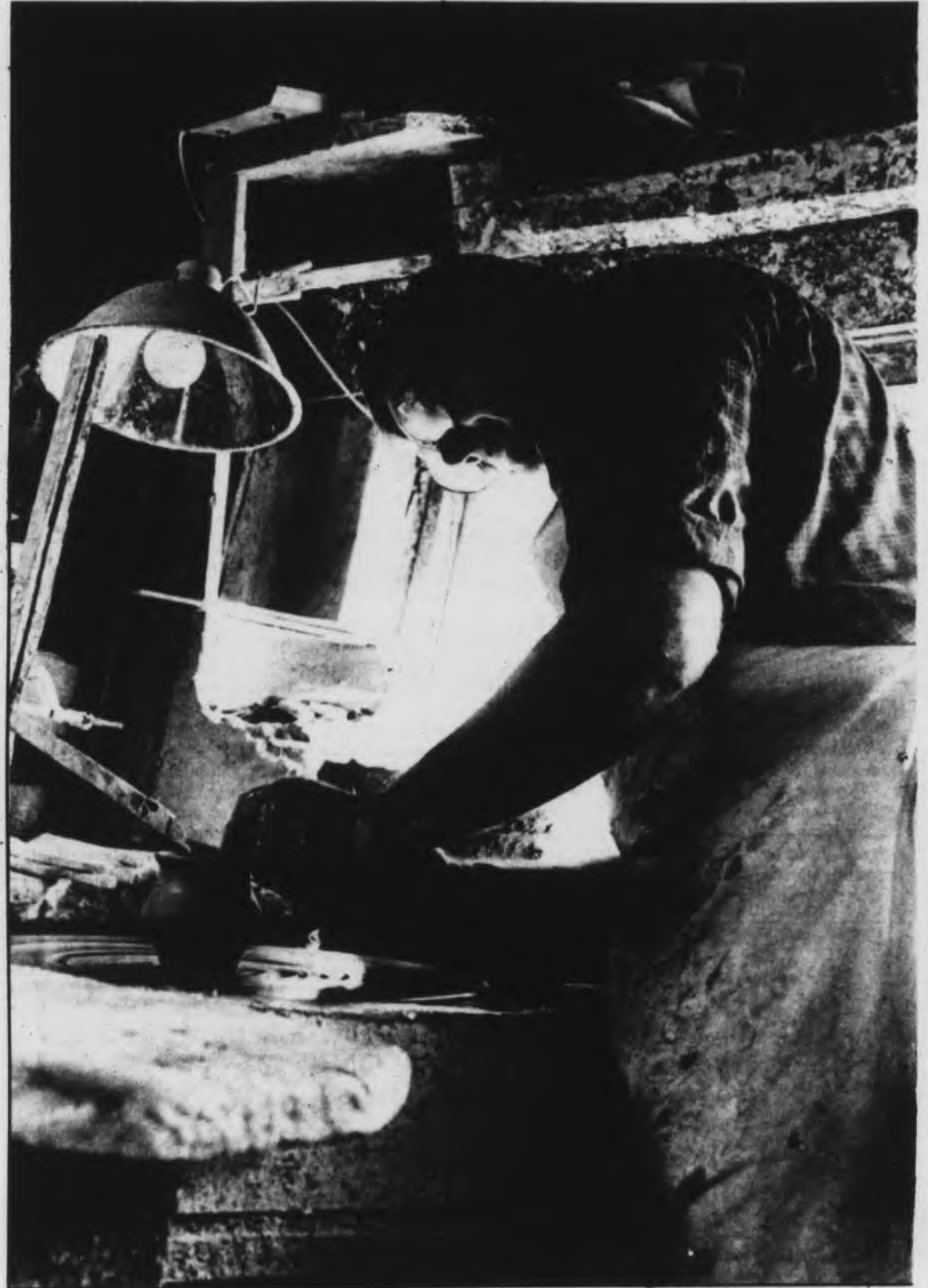
Progress Photo/Charlie Bolton
