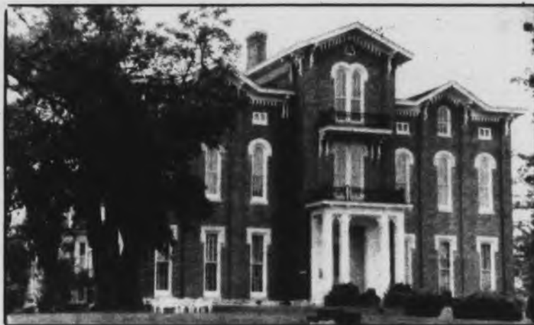
Progress Photo/Leslie Young
