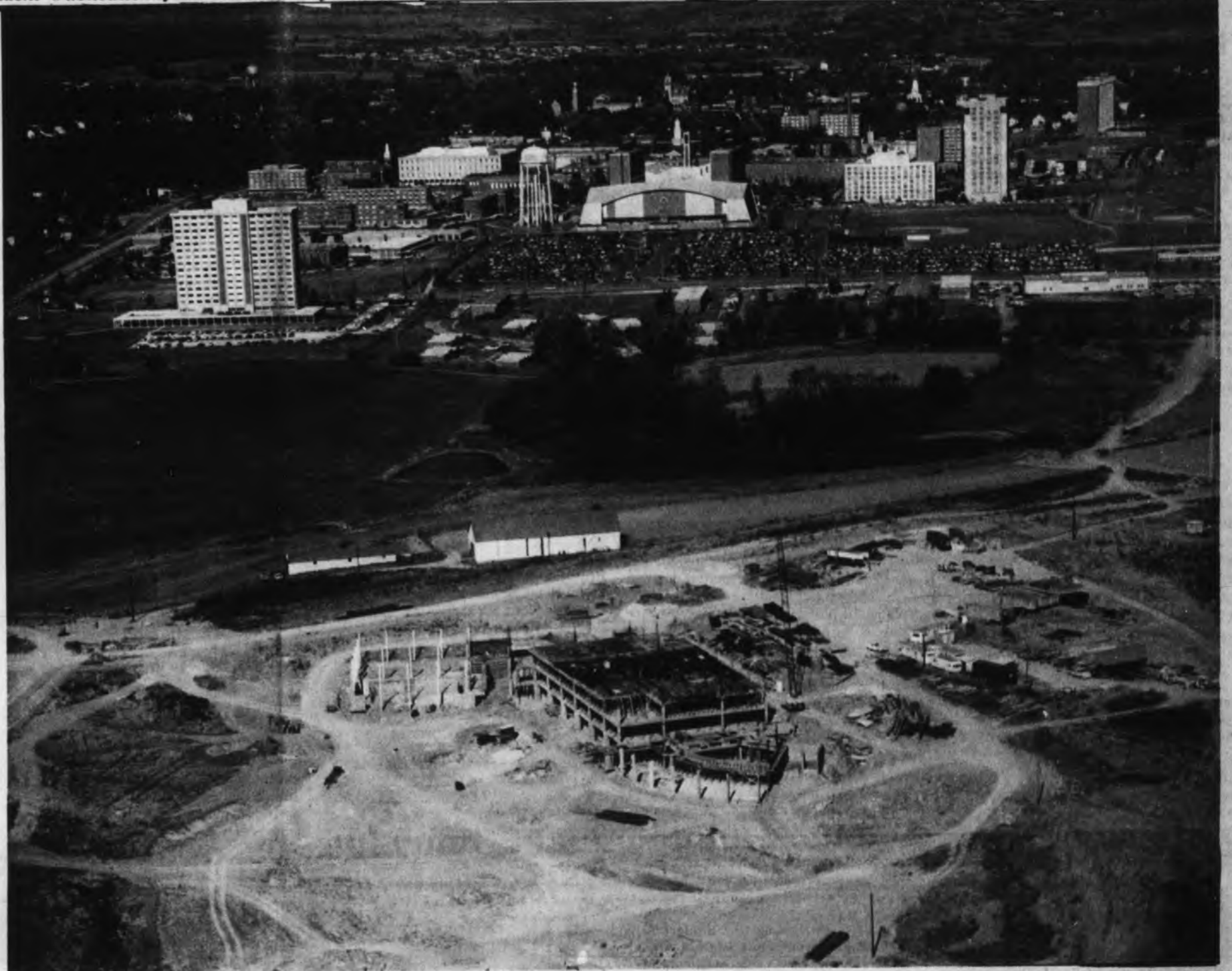
New building takes shape
