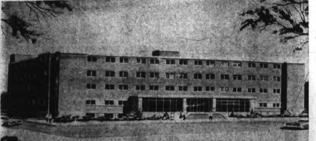
BID AWARDED TO LEXINGTON FIRM FOR WOMEN'S DORMITORY—The Hargett Construction Company, Lexington, was the apparent low bidder on McGregor Hall, six-story women's dormitory to be built at Eastern, it was learned last week.
