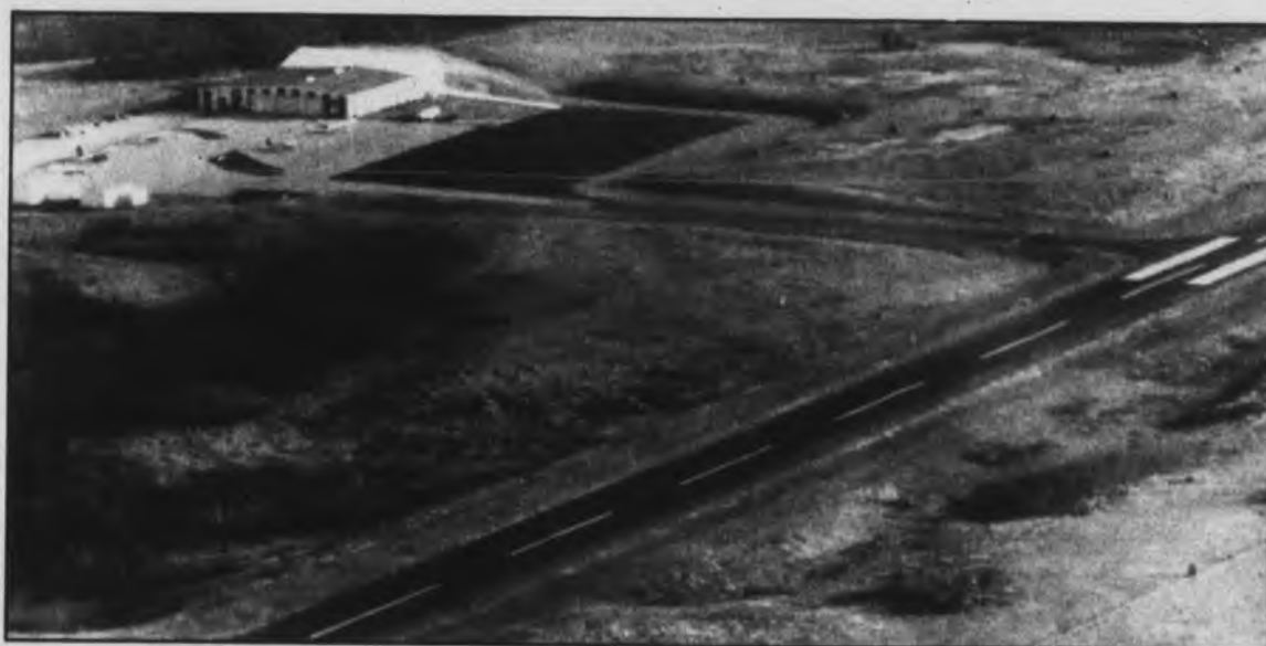
Progress photo by TIM WEBB
