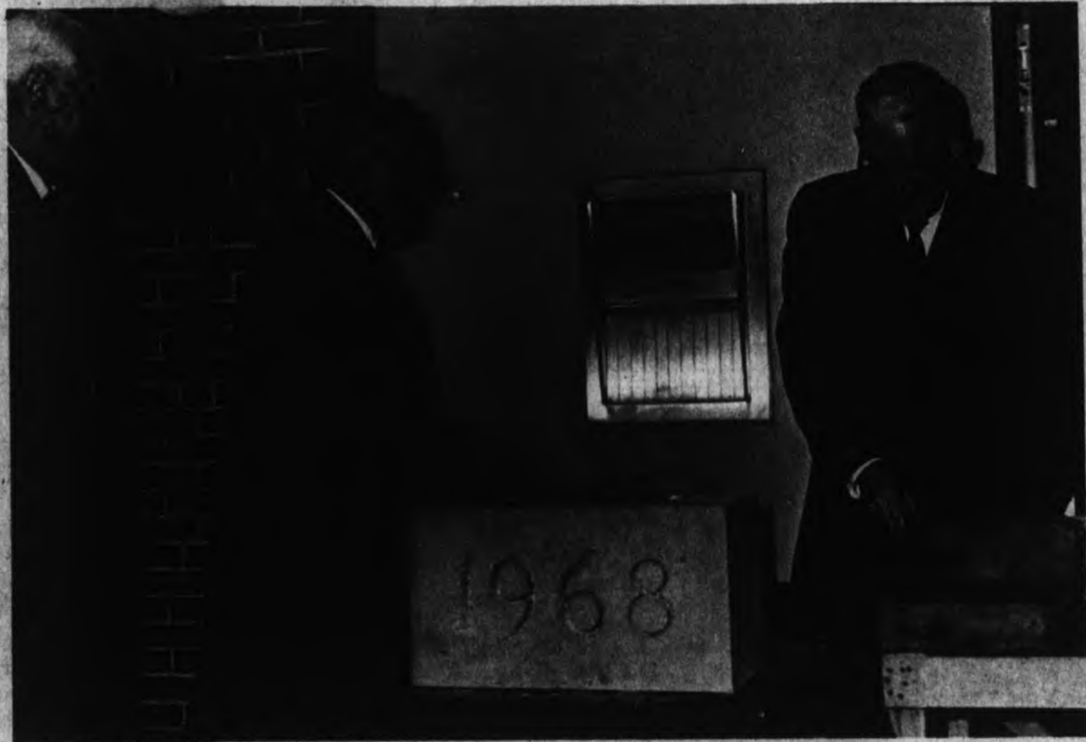
W.C. Jones Lays Cornerstone For Building Bearing His Name
