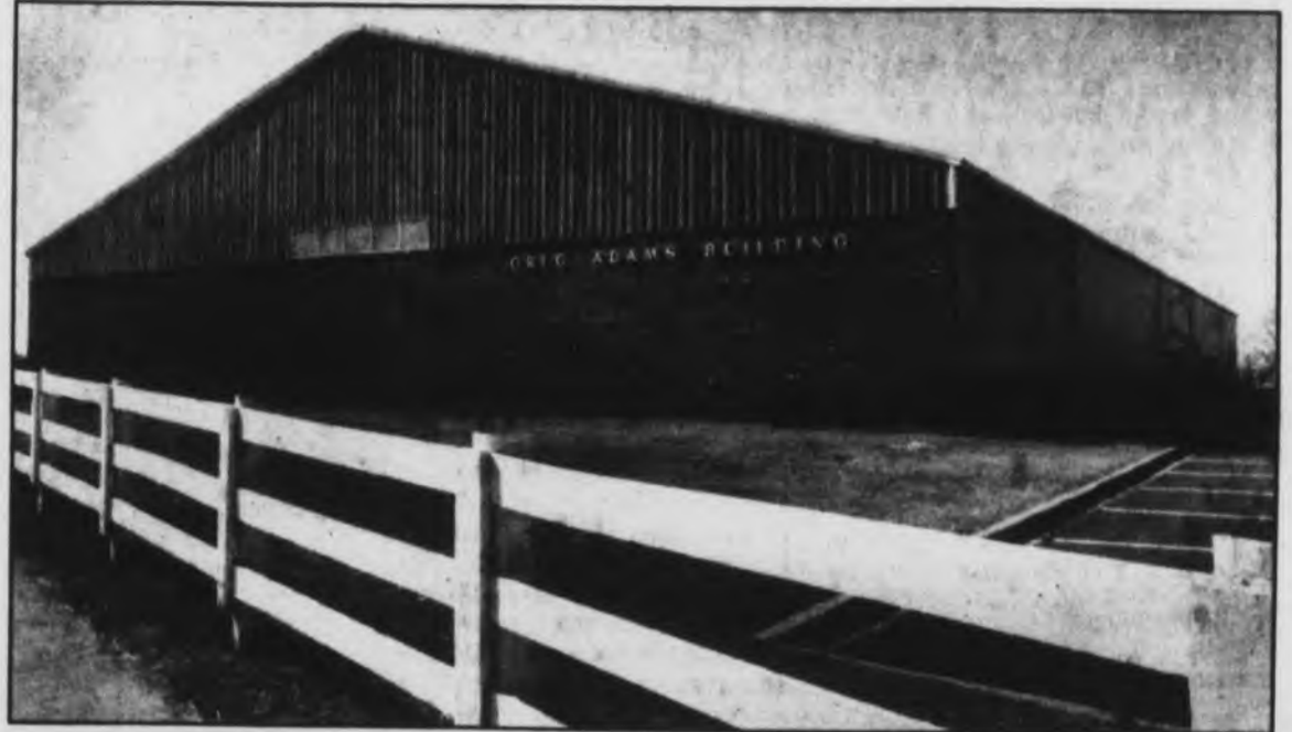
Progress photo by MIKE MORRIS
