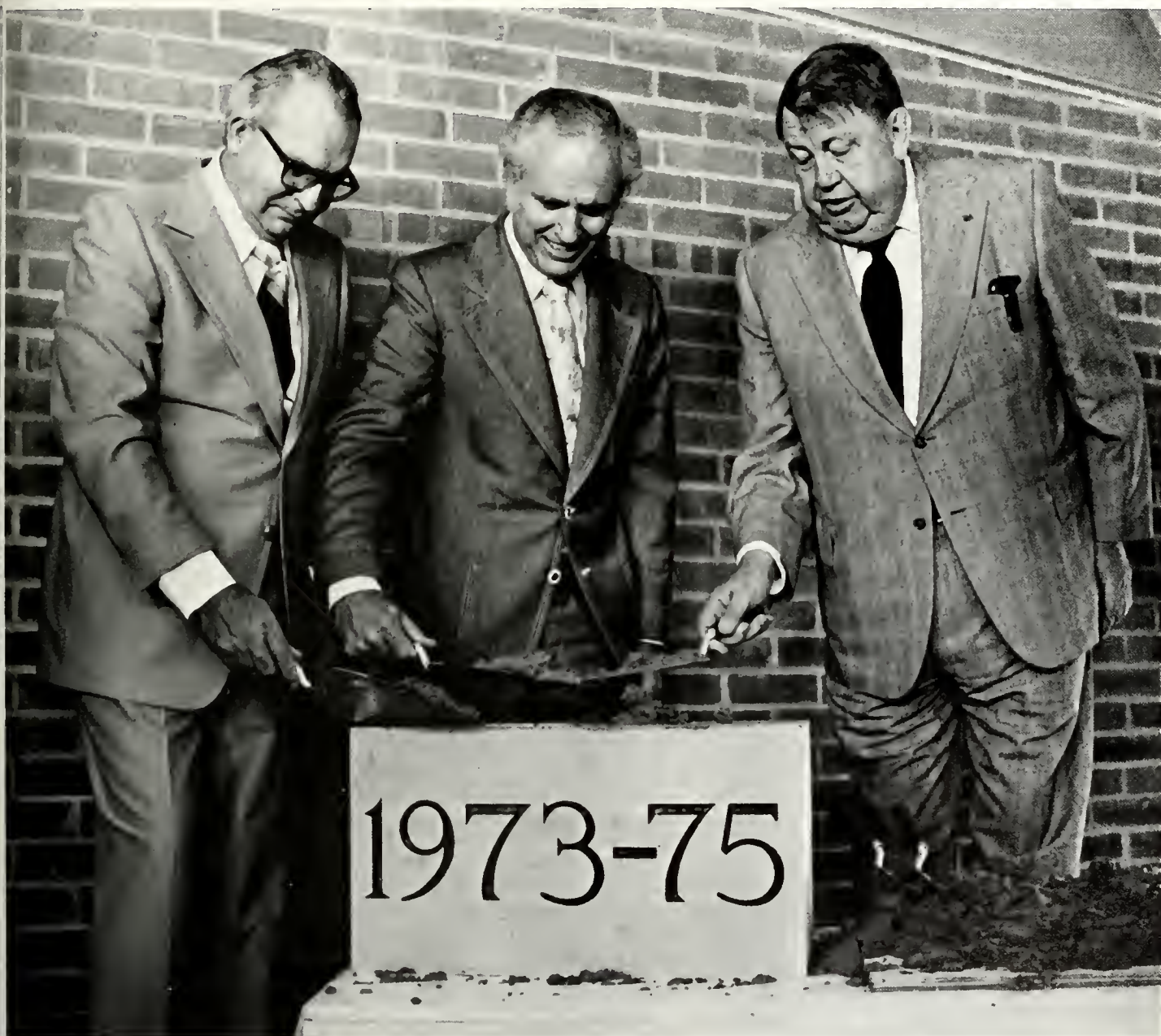
Henry D. Stratton, Governor Julian Carroll and President Martin apply mortar to the cornerstone of the Henry D. Stratton Building, main structure in the Law Enforcement, Fire Science, and Traffic Safety Center.
