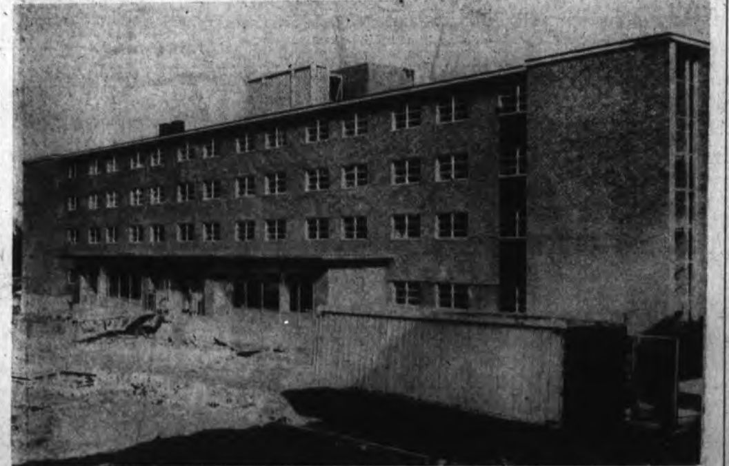
EASTERN DORM NEARS FINISH . . . McGregor Hall, six-story air-conditioned dormitory to house 448 women students, is nearing completion at Eastern. Named to honor Judge Thomas B. McGregor, Frankfort, member of the college board of regents, it will be one of two air-conditioned dormitories occupied this spring at Eastern. The other dorm is Earle Combs Hall, to house 235 men students. Cost of McGregor Hall was $1,958,500.
