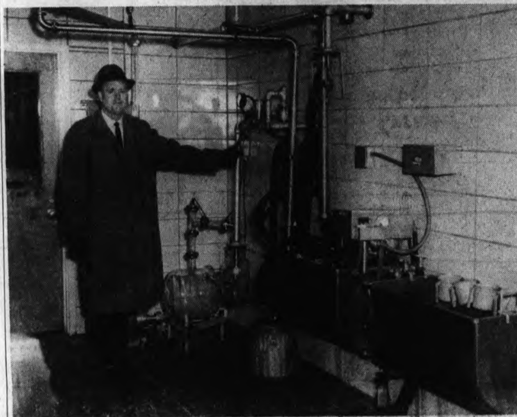
EASTERN'S DAIRY CENTER... Eastern's Stateland Dairy Center, located just across the Eastern State College By-Pass from Alumni Coliseum, is one of the South's most modern dairy facilities. In the top photo the center is shown with its two large silos. In the center photo the 42 cow herd is milked each day. The bottom photo shows assistant professor of agriculture, Mr. Jack Taylor, inspecting the spotless milking parlor. (Bottom photo courtesy of the Richmond Daily Register).
