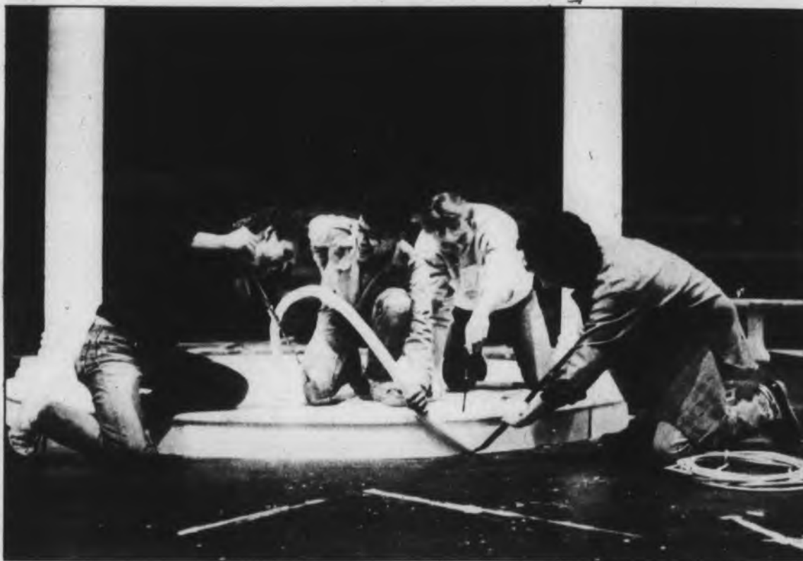
Progress photo/Mike Morris
