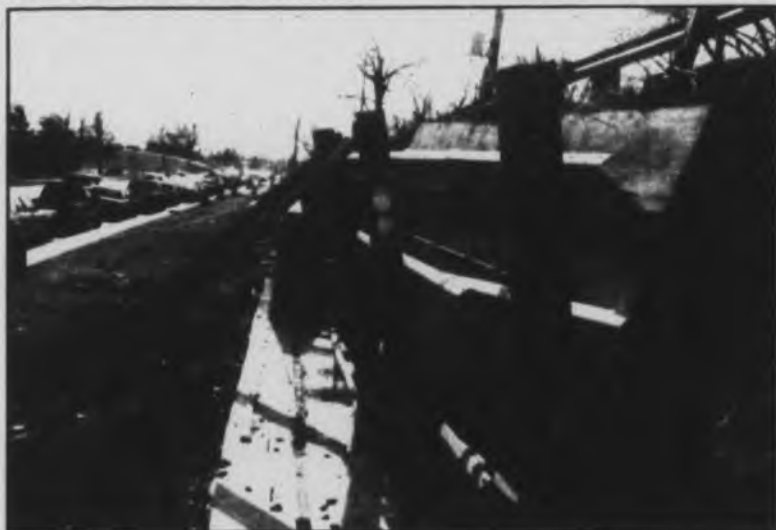
Progress photo by JAY ANGEL
