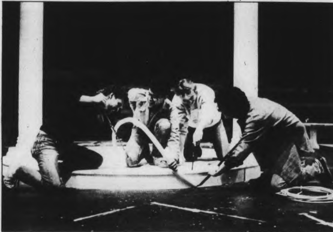
Progress photo/Mike Morris
