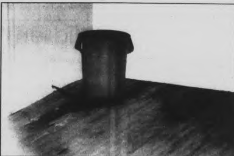
Progress photo by LESLIE YOUNG
