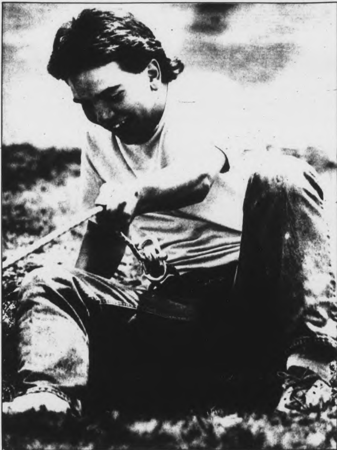
Progress photo/Sean Elkins
