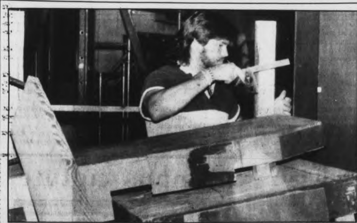
Progress photo by MIKE MORRIS
