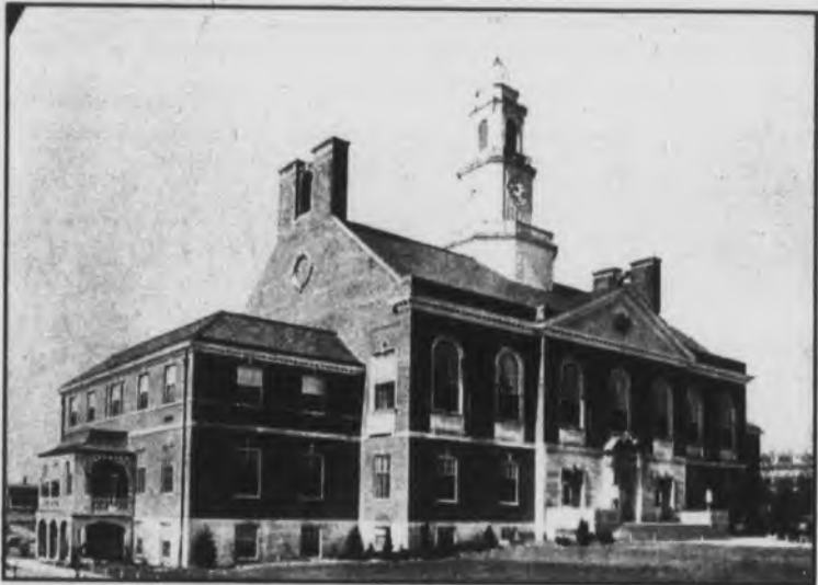
Keen Johnson Building, 1939-40
