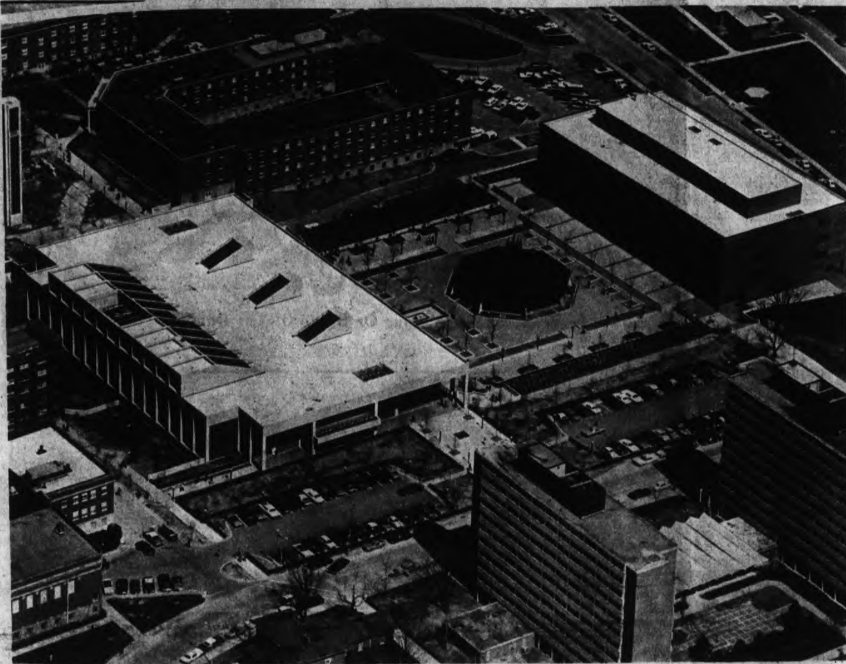
An Aerial View Of The Heart Of Eastern's Campus
