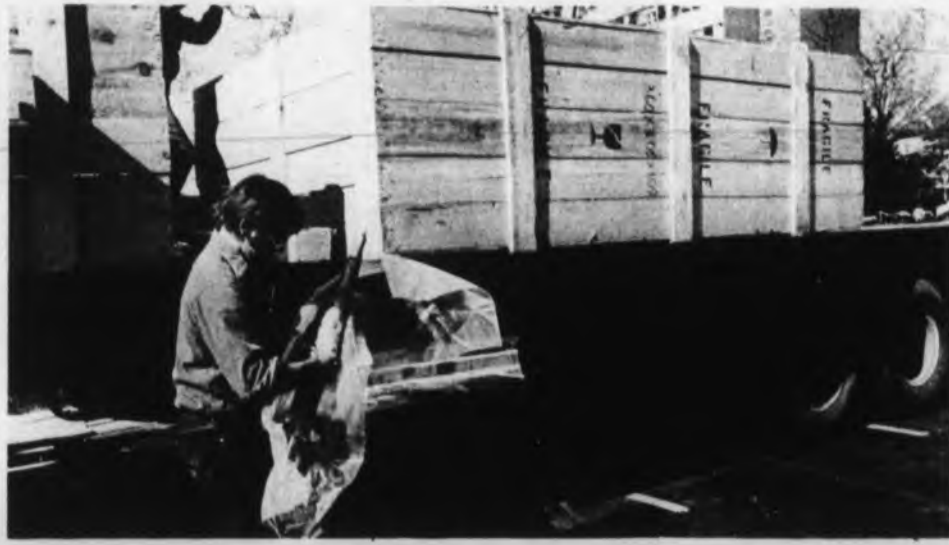
A workman is pictured here unloading one of the final touches to be added to the new statue in the Powell Center Plaza area. The rocket was later mounted in the figure's right hand, while his left hand balanced a sophisticated space craft of the future.
