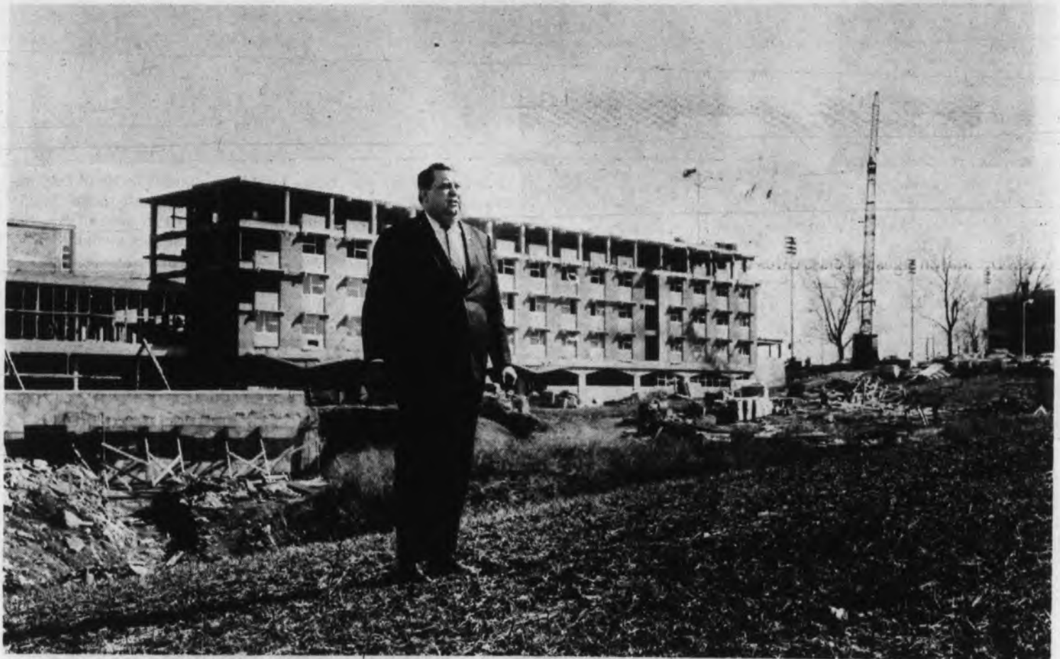
In 1962, President Martin reflects upon the construction of the dormitory named in his honor.
