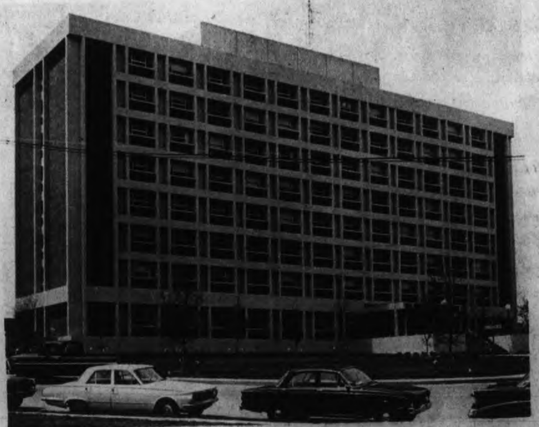
PALMER HALL, AN EIGHT-STORY AIR-CONDITIONED DORMITORY, WAS COMPLETED DURING THE 1965-66 SCHOOL YEAR. THIS BUILDING HOUSES 300 MEN STUDENTS.
