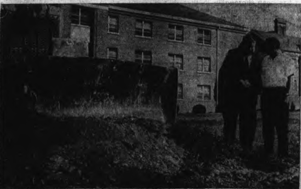
"EARTH MOVING OPERATION" AT EASTERN . . . Construction of a new $2,900,000 classroom building got underway recently as the first earth was turned for the four-story structure. Looking on are President Robert R. Martin, left, and Paul Krambeck, general superintendent of Foster and Creighton contractors, Nashville, Tenn. The air-conditioned building will house the Graduate School and the departments of Business, Education, English and will contain classroom facilities for the simultaneous teaching of nearly 2,200 students. Completion date is expected to be Sept. 1, 1964. See story on page 2.
