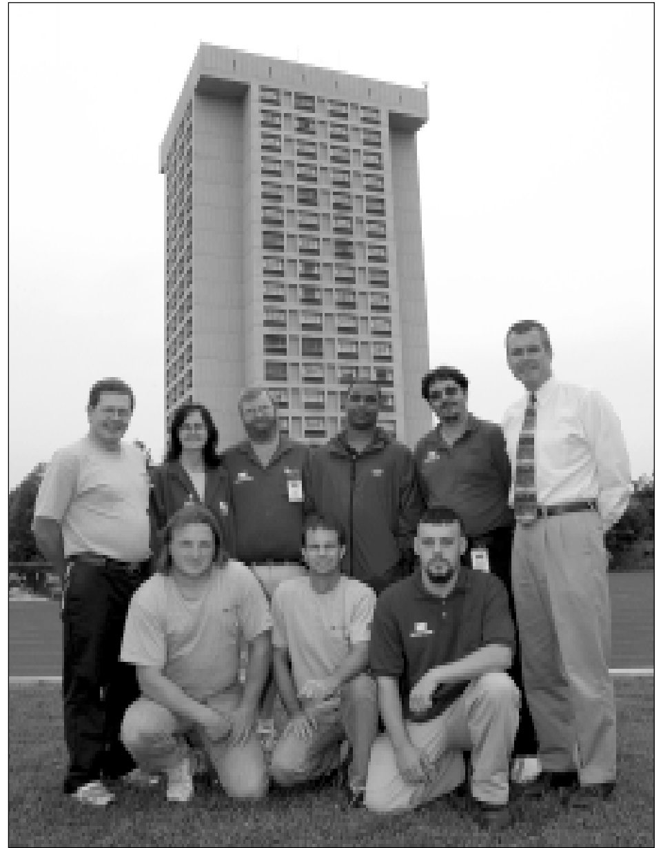
Eight employees of the Division of Facilities Services were given "Beyond the Call of Duty" awards for their recent efforts after a malfunctioning sprinkler flooded portions of Commonwealth Hall. Joining Director James Street, standing far right, are, front from left, Dale King, Frankie Smith, Garney Smith; back row, Melvin Murphy, Rosita Pennington, Ben Pennington, Robert Parks and Everett Woolery. Housing Office employees and other University administrators and employees also assisted in the efforts.
