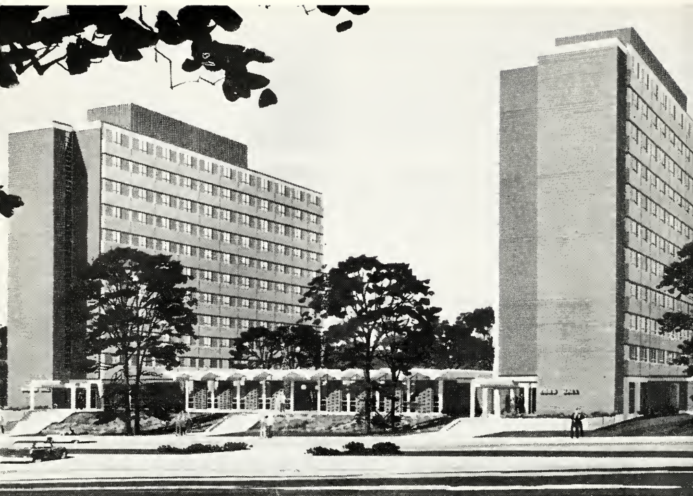
Todd and Dupree Halls, towering 12-story, fully air-conditioned men's dormitories, will house 360 students each when completed in Sept. 1964.
