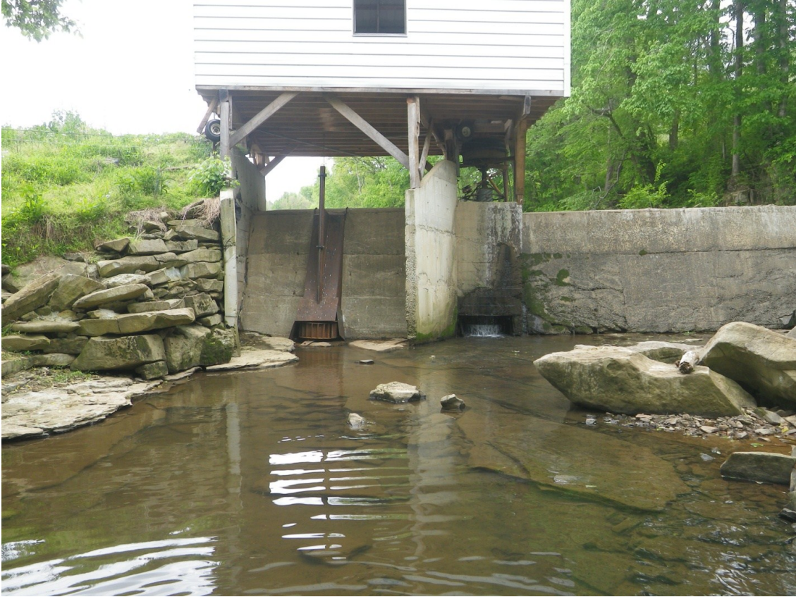
Figure 7. Concrete impoundment for a saw mill operation, encountered during sampling efforts at Pinchgut Creek, Allen County KY (36.65726 -86.02689).
