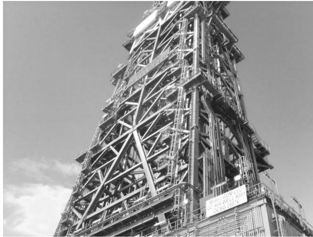
Figure 2. Rig's Dual Derrick
